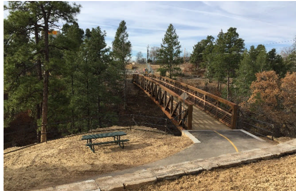
Figure 4: CANYON RIM TRAIL PHASE II BRIDGE
