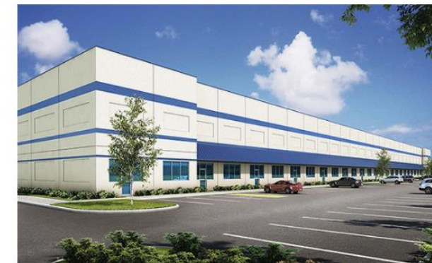
This 85,000 square foot flex warehouse, located on the east side of Baltimore, Maryland, was designed as a shell to meet LEED Silver and Baltimore's Green Building Standards. Photo Credit: Arium | AE
