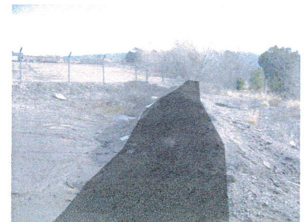
The trail could replace existing stormwater controls and serve to channel and detain surface runoff.
