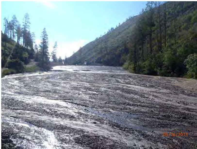
Figure 4.34. Sediment Filled Reservoir
