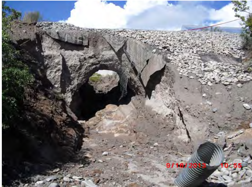
Figure 4.25. West Holding Pond at Pajarito Cliffs Site
