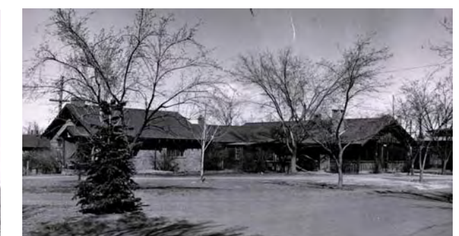
1935 Stone addition to Spruce Cottage for Master Counselor for Spruce Troop designed by John Gaw Meem in "Rustic" NPS Style with Bungalow Influences encroach into green.
