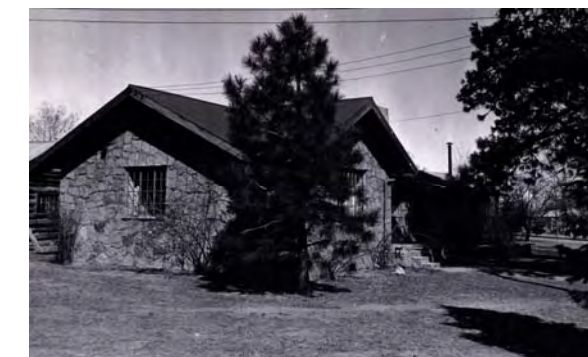
Stone addition to Guest House built in 1935 by John Gaw Meem; "Rustic" NPS Style with Bungalow influences
