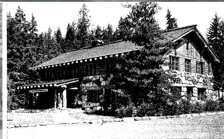
Administration Building, Longmire, Mount Rainier National Park
