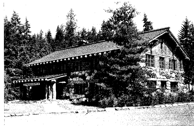
Administration Building, Longmire, Mount Rainier National Park
