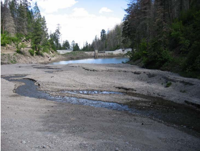
The Los Alamos Reservoir has been severely impacted by two wildfires
