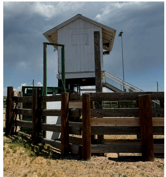
South side of Announcer's box structure
