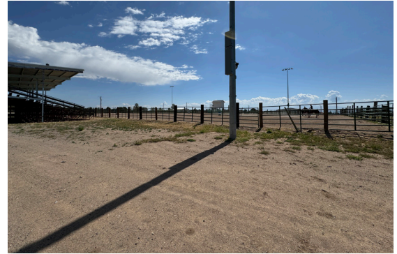
West view of Project Site
