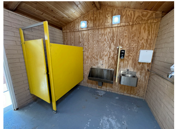
Interior View of Restrooms
