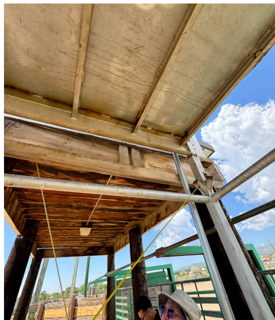
View under Announcer Box structure
