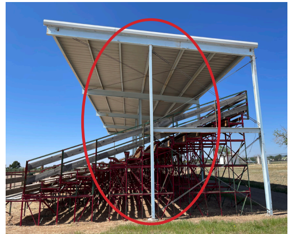
View of bending column
