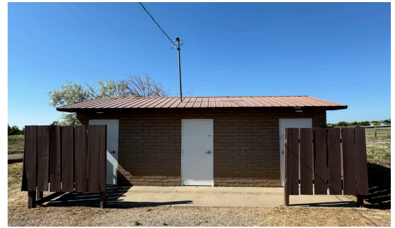
North side of Restrooms
