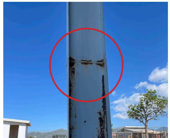
View of column welds
