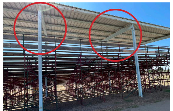
View of lateral web bending
