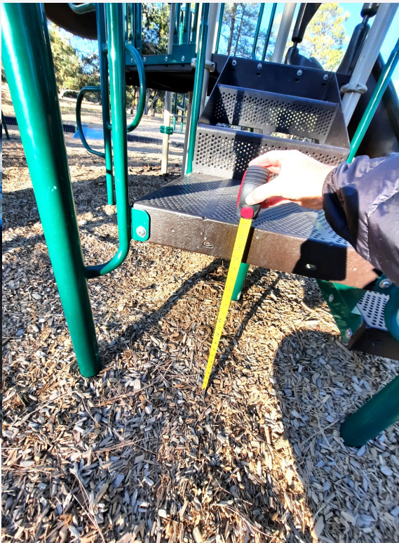
Transfer system installed incorrectly
