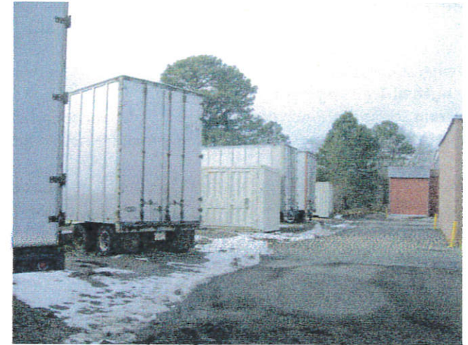
Once existing storage trailers are relocated, construction of the short A-2 segment will be easy.
