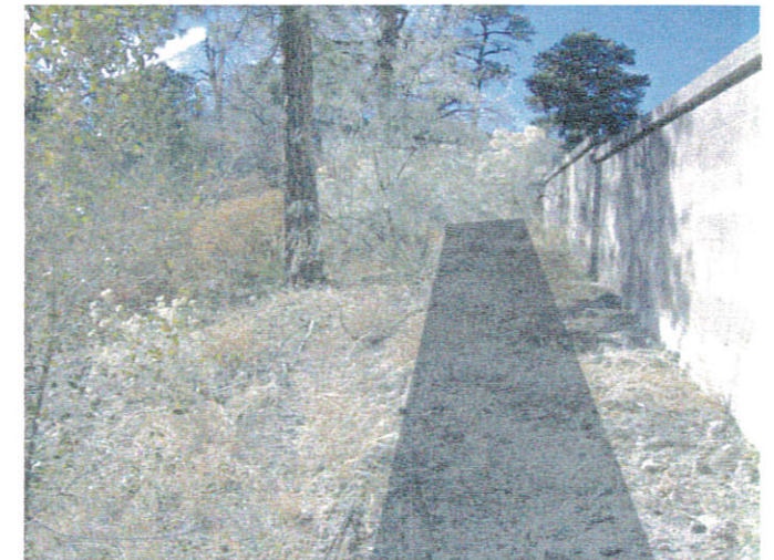
The west half of the parcel is relatively flat.
