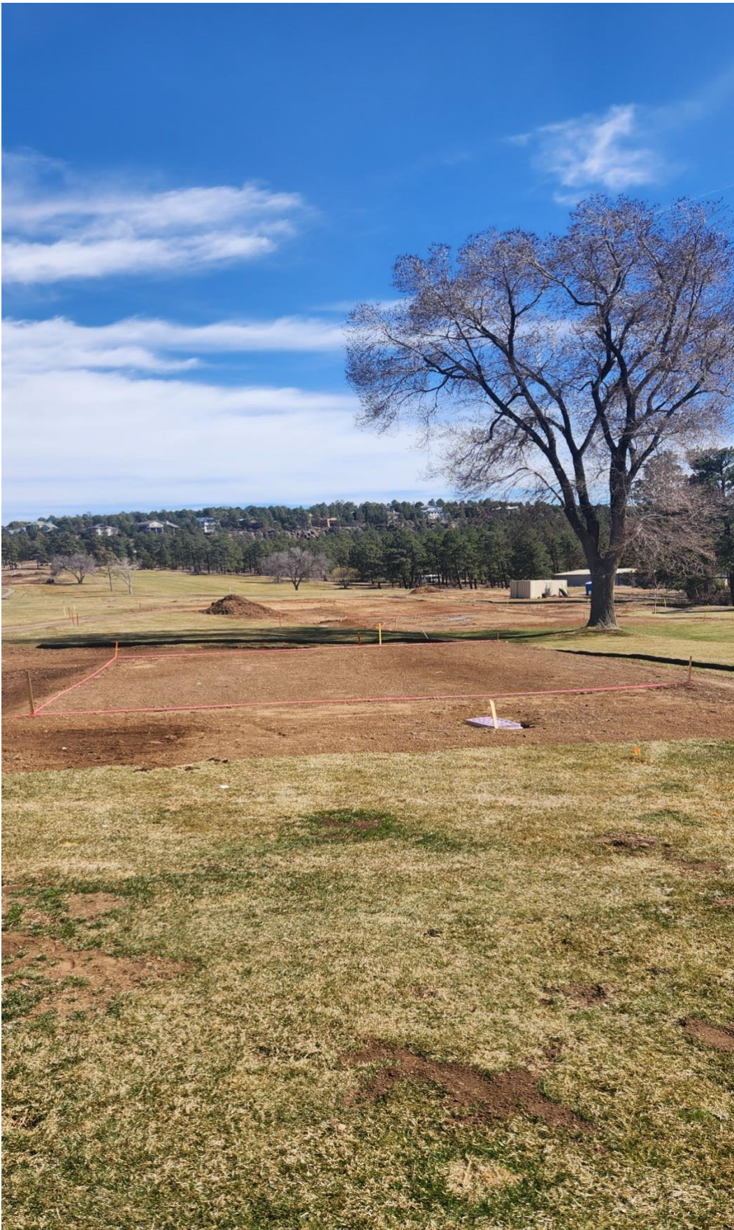
HOLE #5 NEW TEE COMPLEX, VIEW FROM NEW BACK TEES
