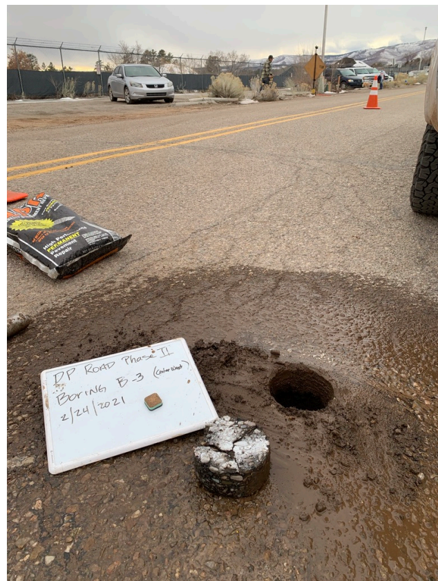
Boring B-3 After Coring
