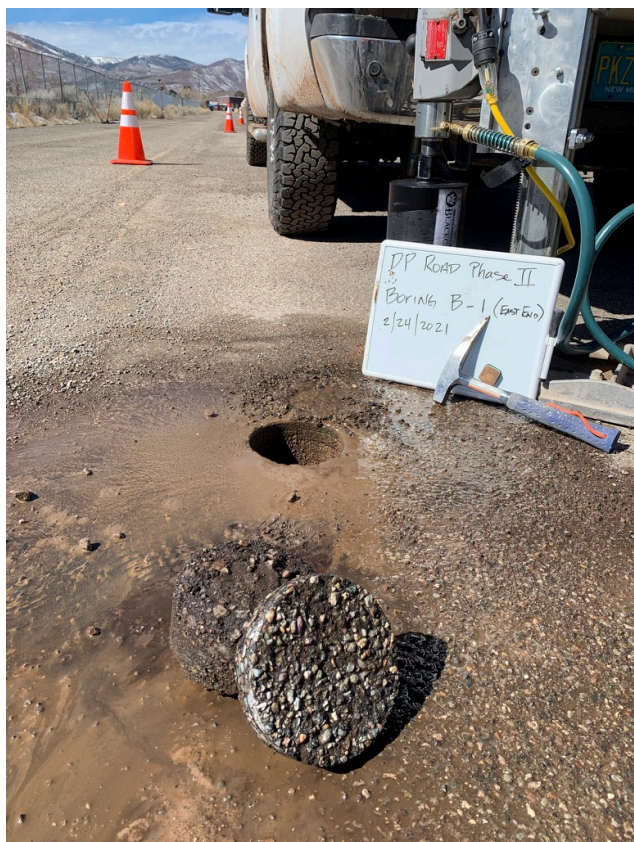
Boring B-1 After Coring
