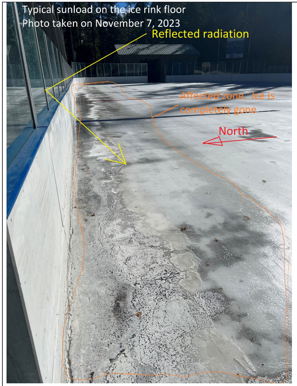
Figure 1. Typical sun load acting on the ice rink floor during the late October to December period. The image shows the north edge of the floor. This is the most impacted area on the floor. Image taken on November 7, 2023, at 9:48 am by Brendan Tuning, Los Alamos County ice rink operator.
