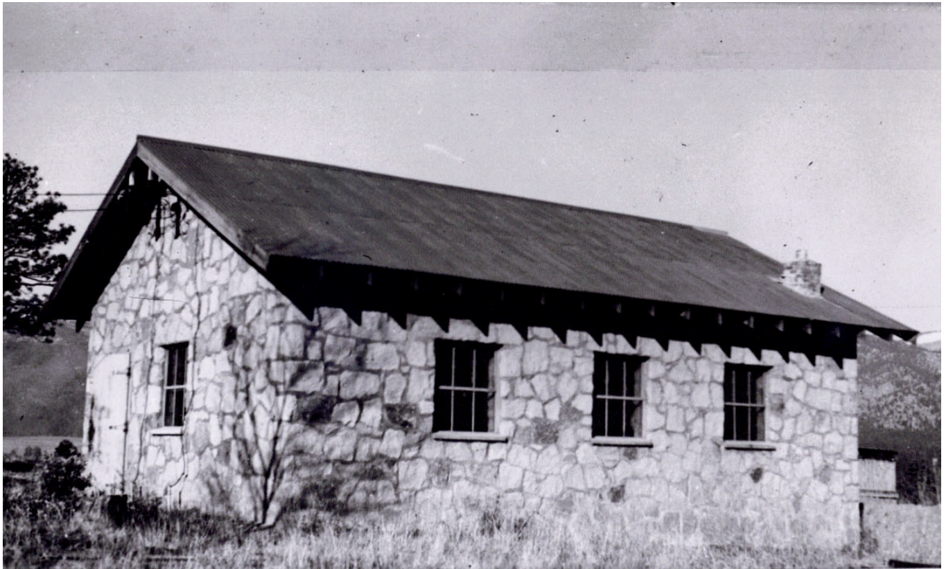
LARS Power House 1942. Photograph courtesy of Los Alamos Historical Society
