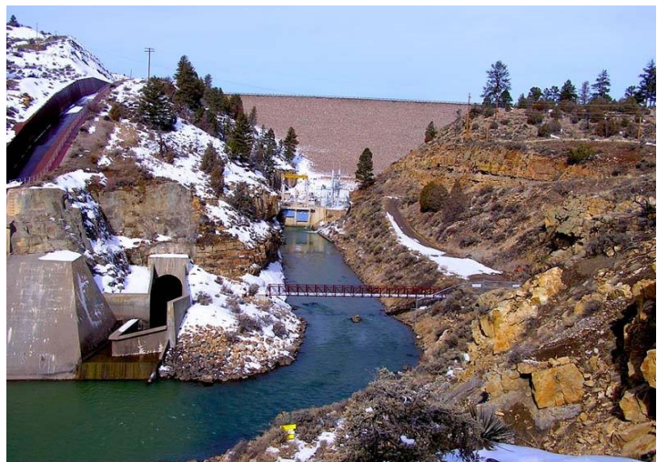
El Vado Hydroelectric Power Plant
