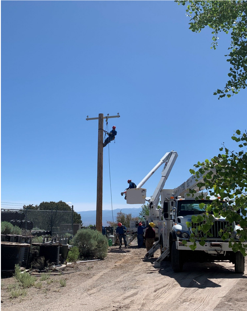
The Electric Distribution Division participates in overhead system safety training.
