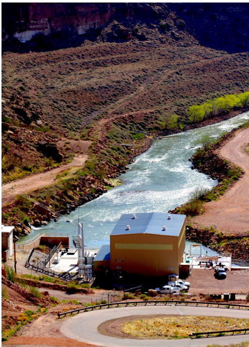
Abiquiu Hydroelectric Power Plant
