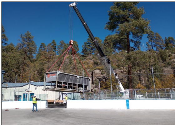
Installation of temporary chiller at the Ice Rink
