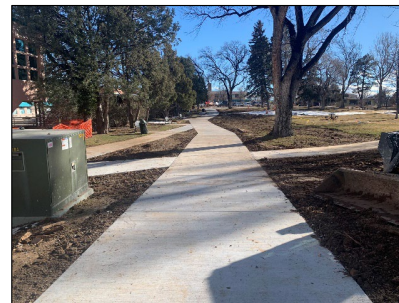
Urban Trail Construction Project
