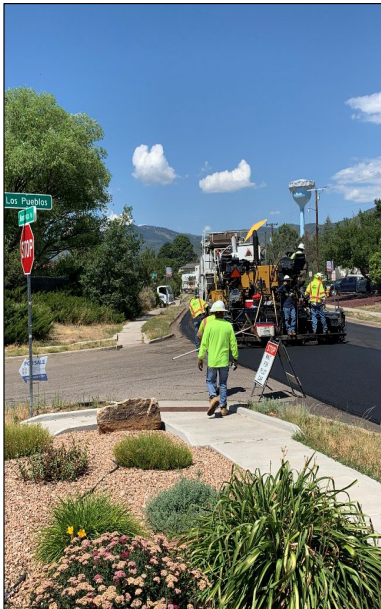
Barranca Mill & Overlay Project
